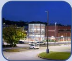
Low Bay, Gymnasiums, Warehouse, Site & Area
